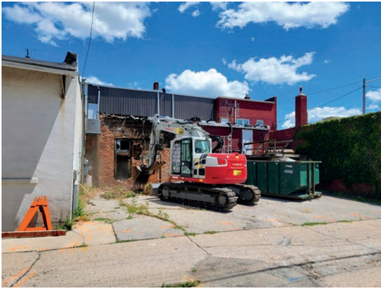
Demolition has begun in the alley behind 4 and 6 First St. NW, the former Rick's Pharmacy building.
