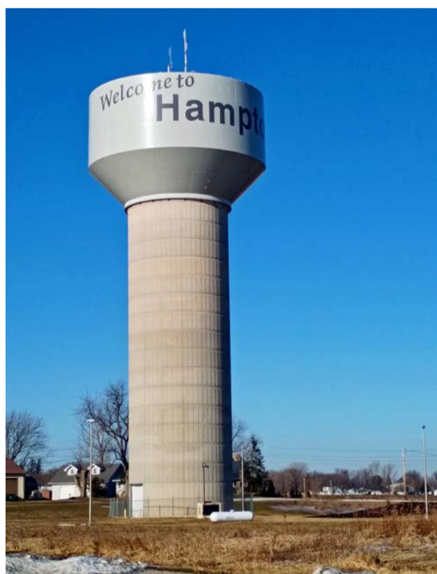
The City of Hampton recently renewed a lease with a phone company who is renting space on their water tower for internet equipment.
